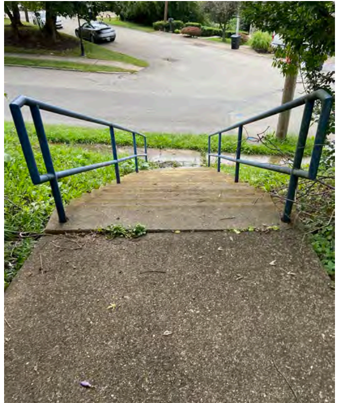
Linwood Park is only connected to the sidewalk by stairs.
