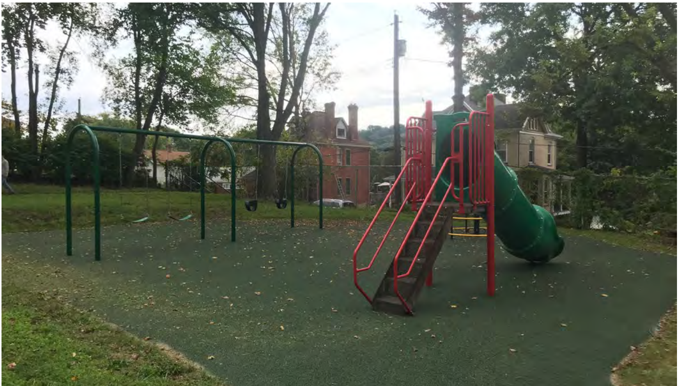
The existing rubber safety surfacing is an accessible option for play areas.
